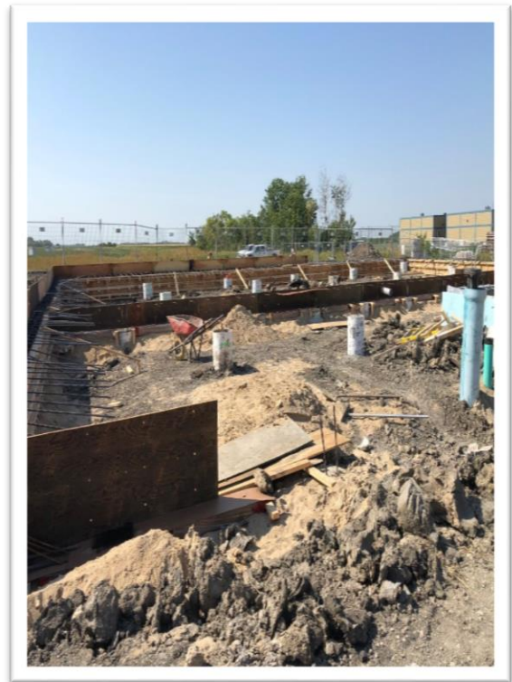
Forming of beams and footing
