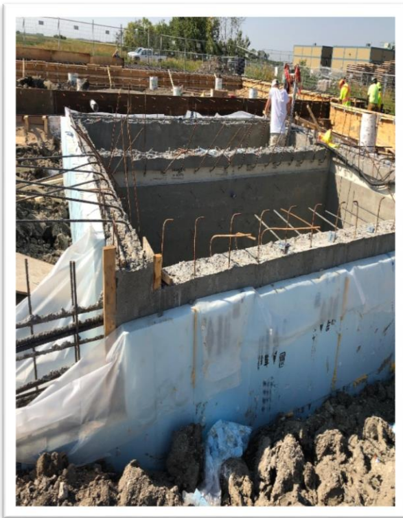
Cistern completed and insulated
