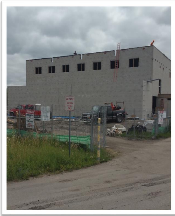
North side of Gym wall
