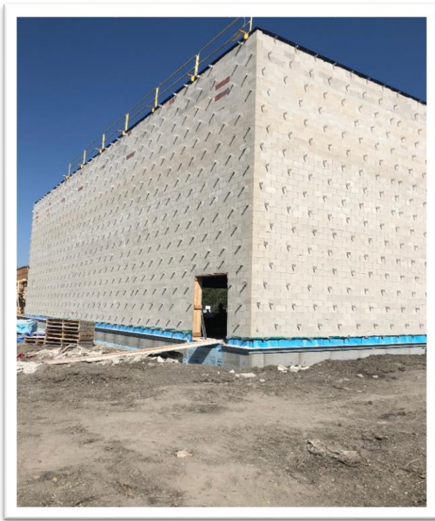
Gym exterior complete – roof deck installed and sealed
