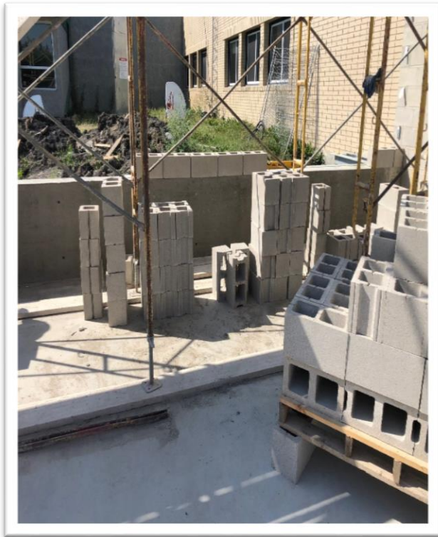
South classroom exterior wall being constructed
